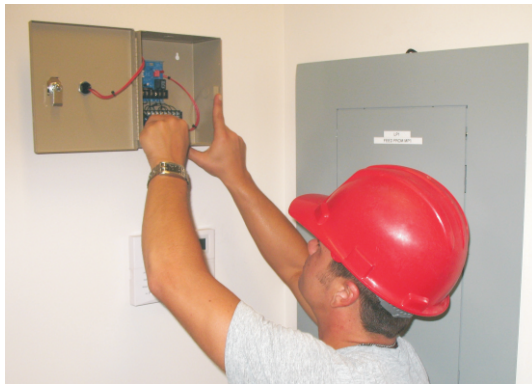
Dedicated terminals on the logic panel facilitate easy wiring. Auxiliary terminals can also be wired to a central alarm system.
