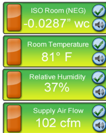
Fig 5. Quad Station View
